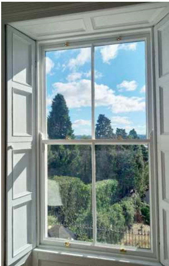
Figure 45: Two-over-two pane timber sash window
