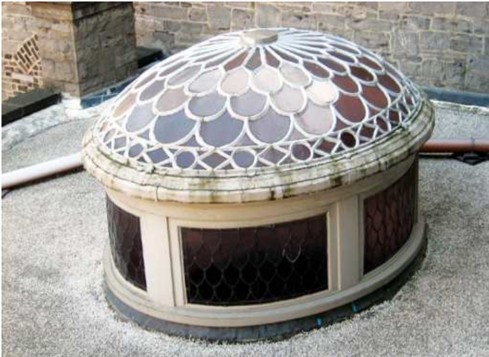
Figure 37: Historic skylights and lanterns, such as this fine example, should be well maintained but can be difficult to upgrade thermally. Consideration should be given to adding secondary glazing at ceiling level (Image from Advice Series: Energy Efficiency in Traditional Buildings , 2010)
