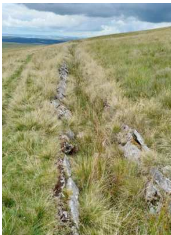
Figure 68: Disused gravity fed water channel for a hydro scheme
