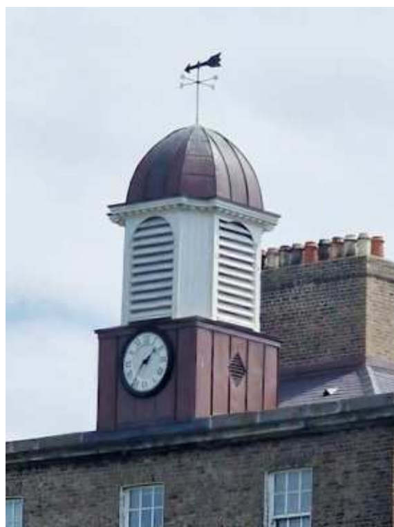
Figure 60: Copper-covered dome over louvred timber vent
