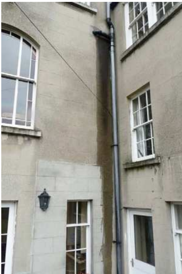
Figure 24: Example of cement render applied to a traditional building
