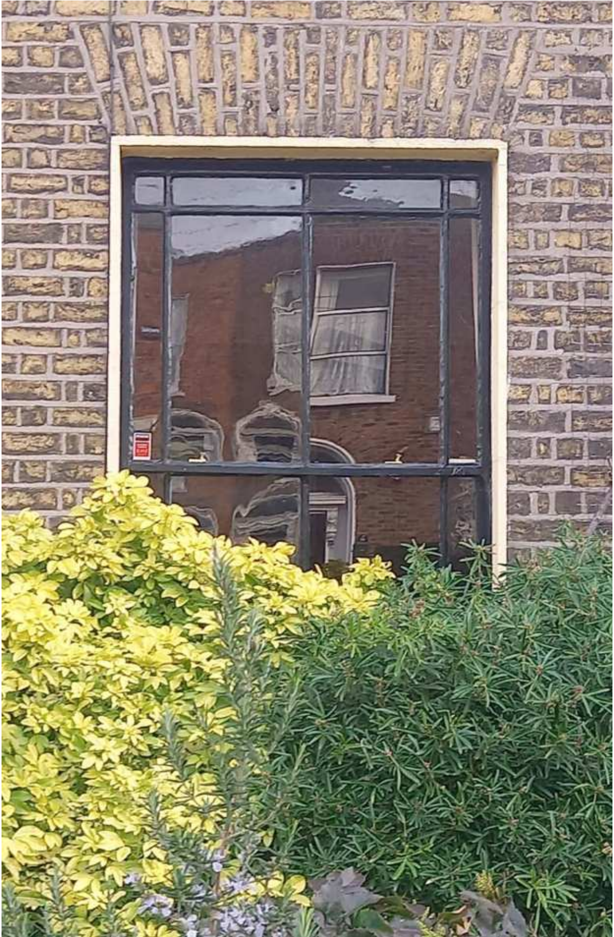
Figure 44: Timber sash window with original glass panes
