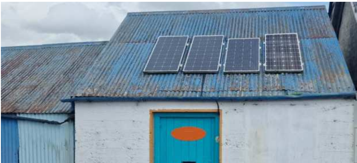
Figure 67: PV on the roof of an outbuilding
